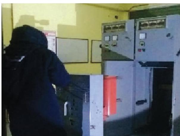
▶▶▶ Kerja-kerja penggantian Single Busbar Air Insulated Vacuum Switchgear 11KV di FINAS Petaling Jaya.
